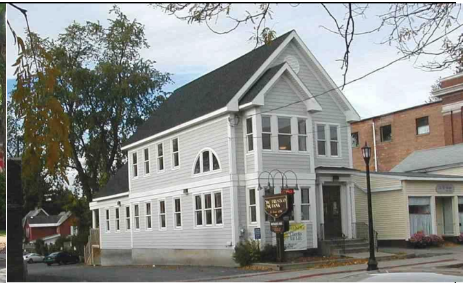
This property was originally intended to be removed to construct a new one. Instead, extensive renovations were made to the building so it would blend in with the existing streetscape.
